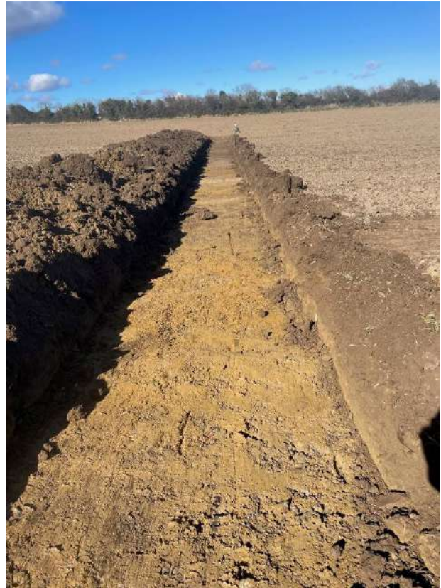
Plate 10 Trench 14, facing north-northwest
