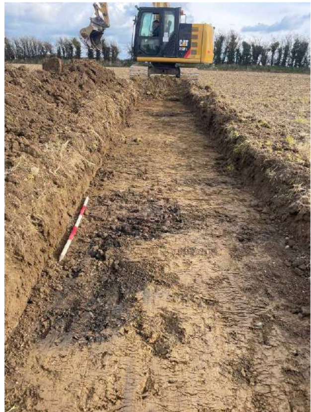
Plate 4 Trench 4, facing northeast, burnt spreads 4.1/4.2
