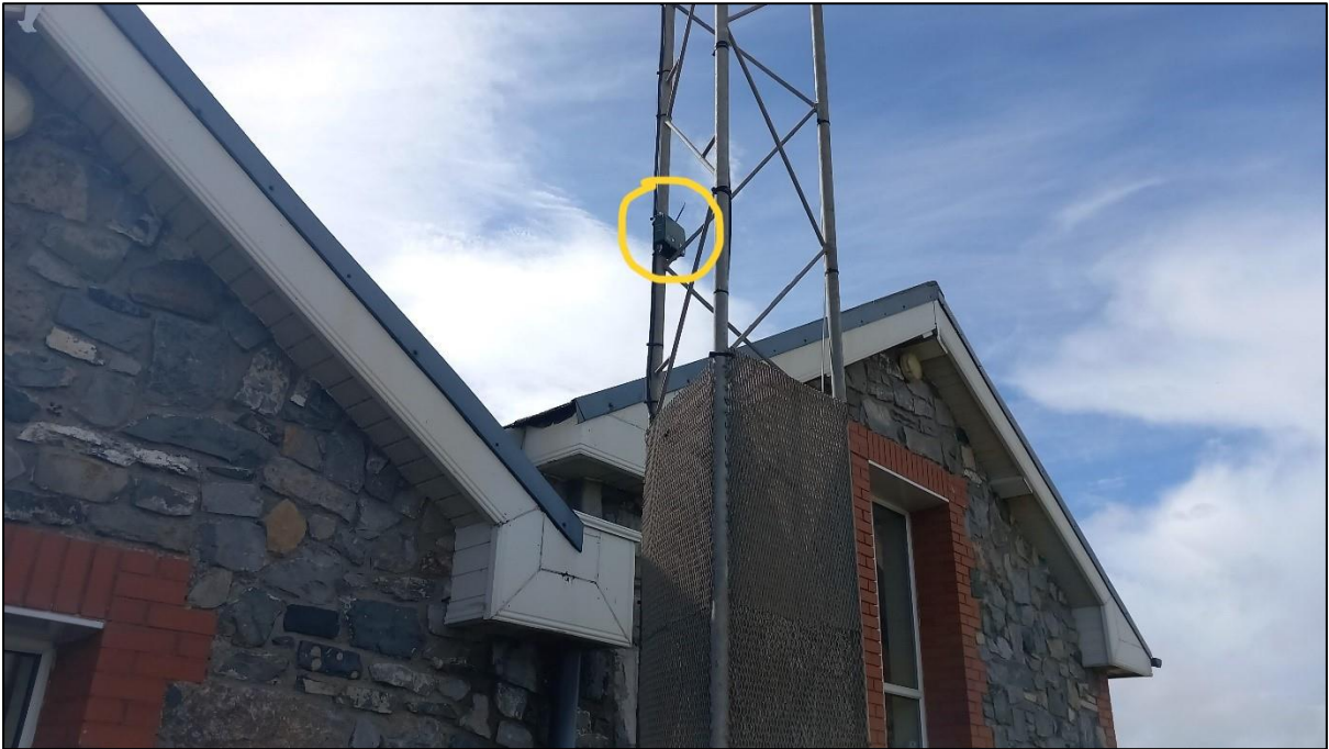
Plate 3 - Skerries detector on the RLNI weather mast detector circled in yellow (integrated mic)
