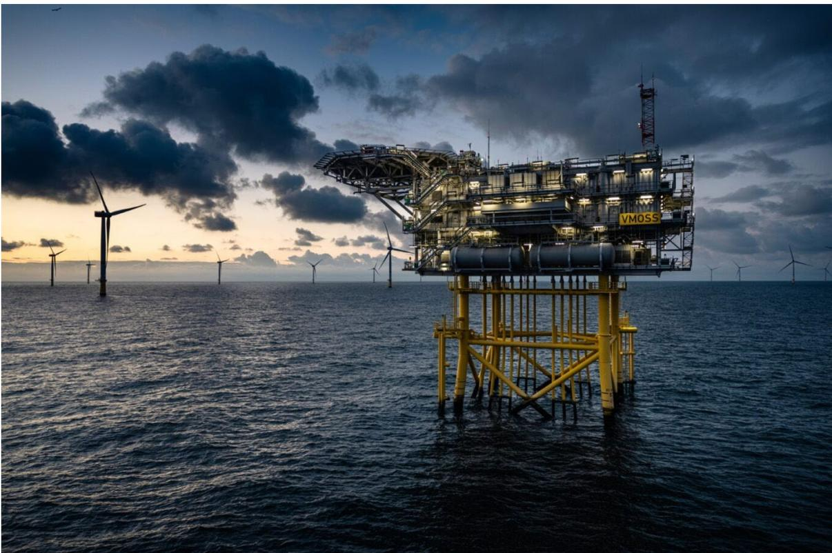
**Image 6.5 Typical OSP on jacket foundation (Source: CIP – Veja Mate)**
