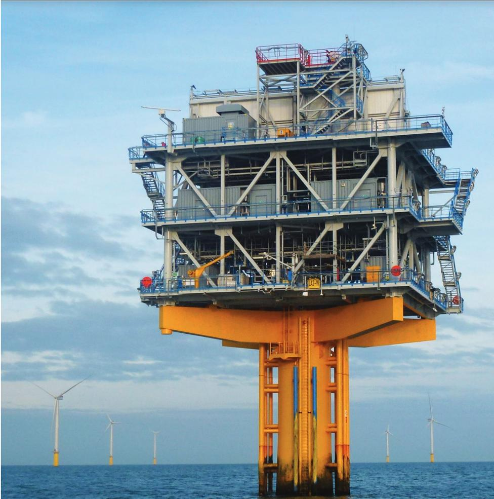
**Image 6.4 Typical OSP on monopile foundation (Source: Arup)**
