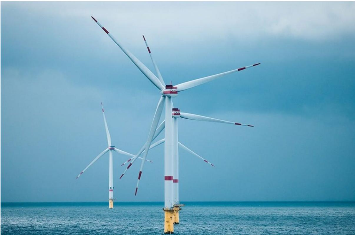
**Image 6.6 Typical WTG on a Monopile foundation (Source: CIP)**
