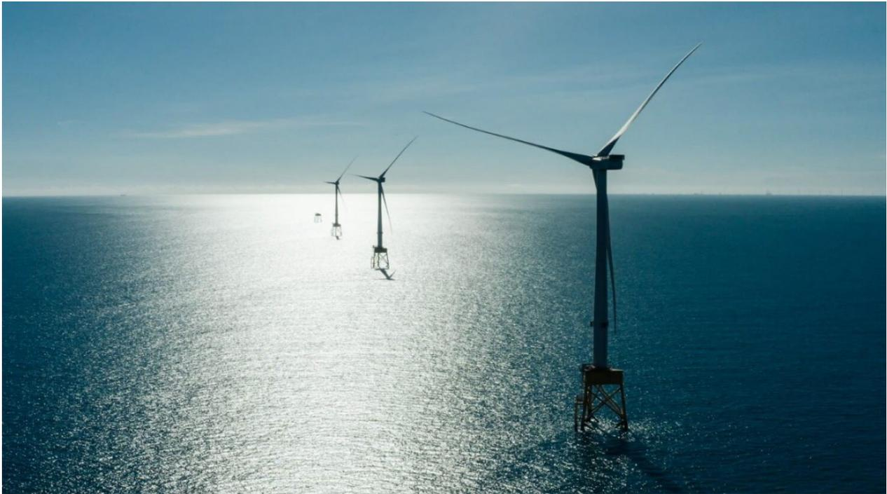
**Image 6.7 Typical WTG on a Jacket foundation (Source: CIP)**
