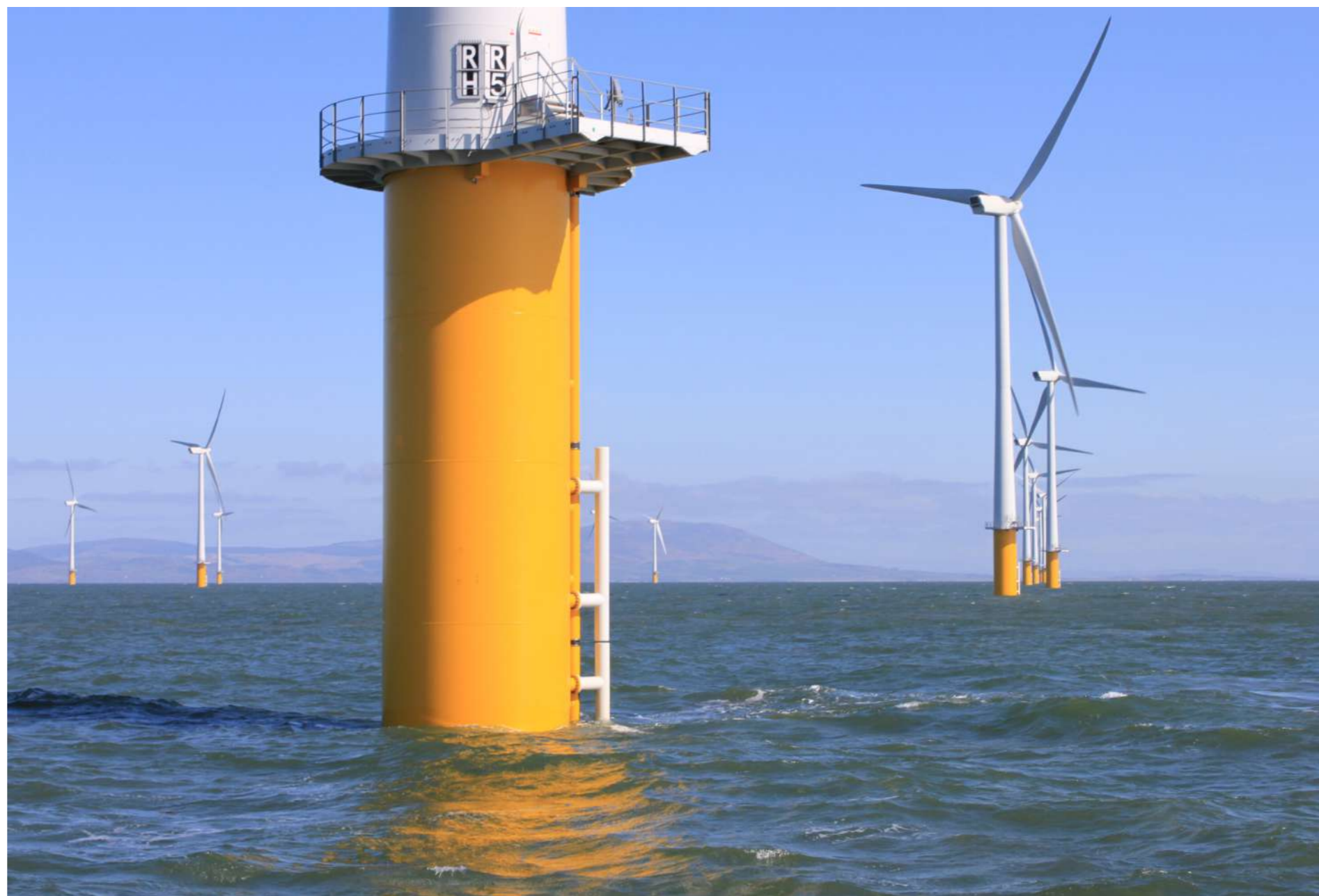
Image 6 Typical WTG on a Monopile foundation (Source: Arup)
