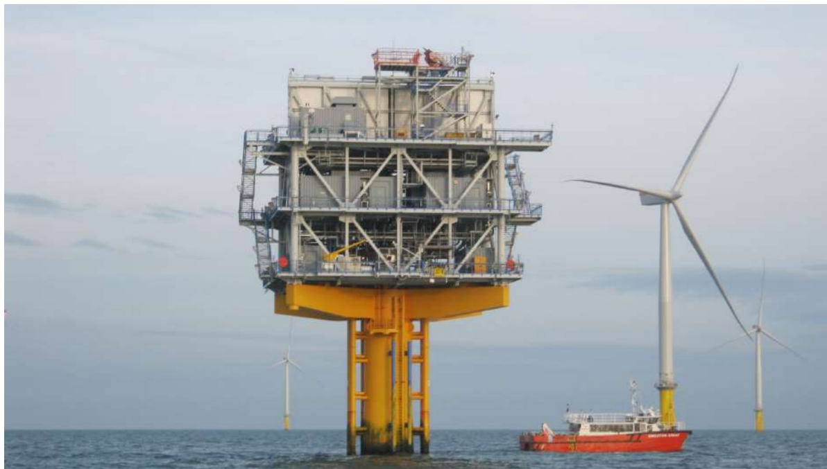
Image 5 Typical OSP on monopile foundation (Source: Arup)
