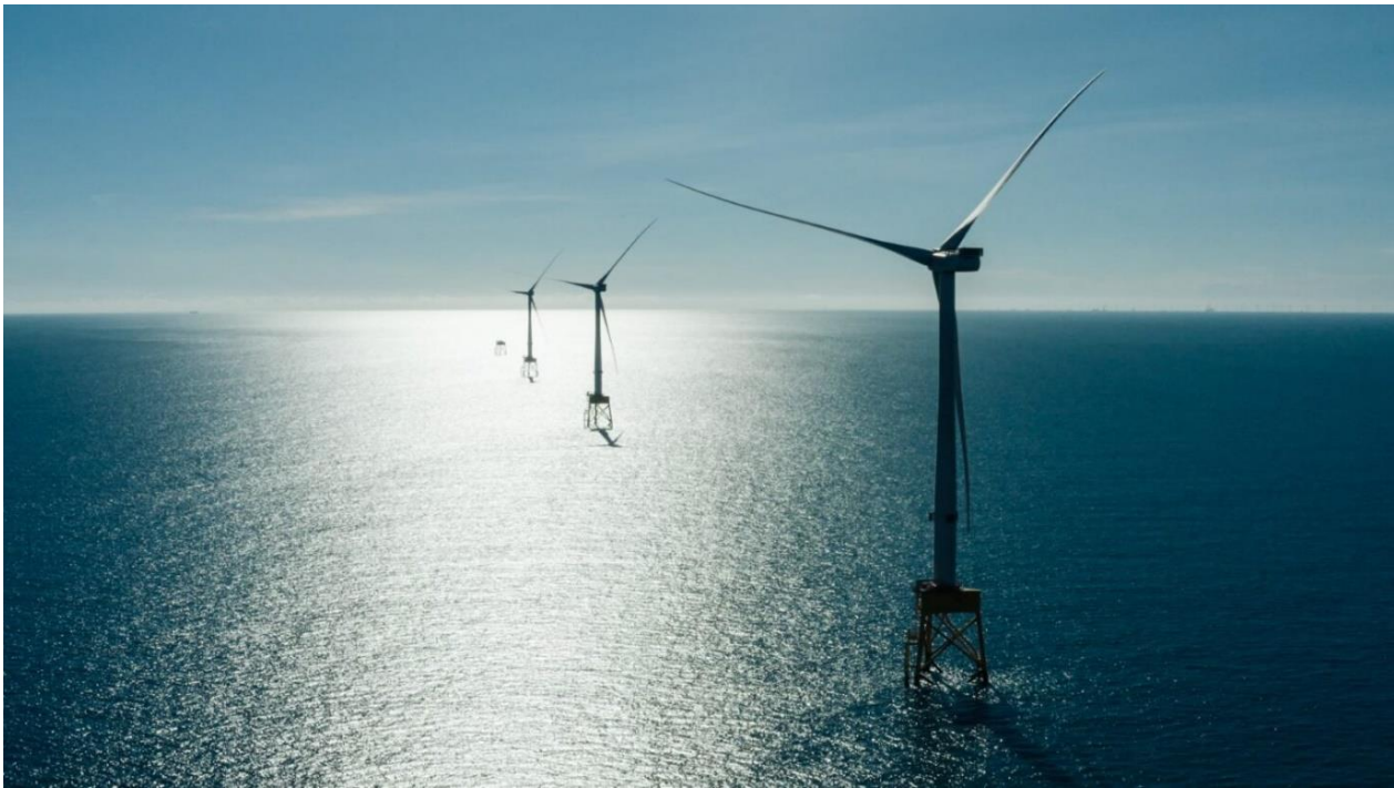
Image A6.2 Typical WTG on a Jacket foundation (Source: CIP) (Replacing Image 6.6 of the 2024 EIAR)
