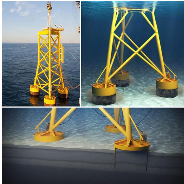
Figure 3.3 Suction Bucket Jacket Foundations
