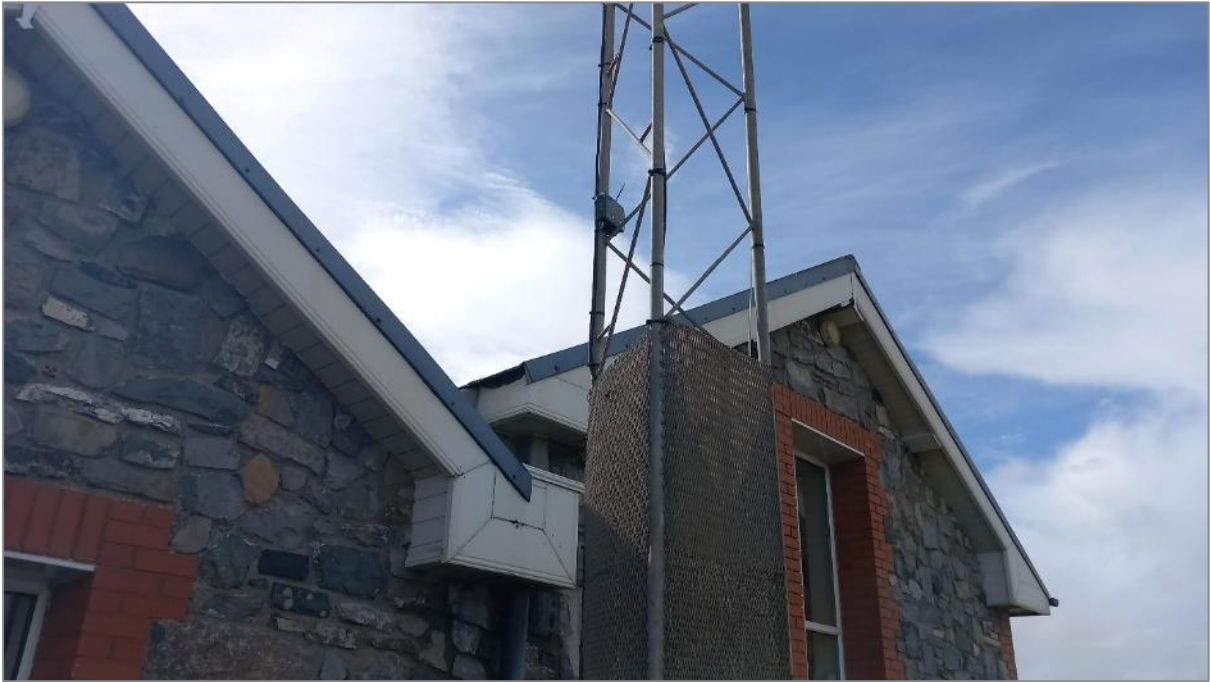
Plate 3: Skerries detector on the RNLI weather mast
