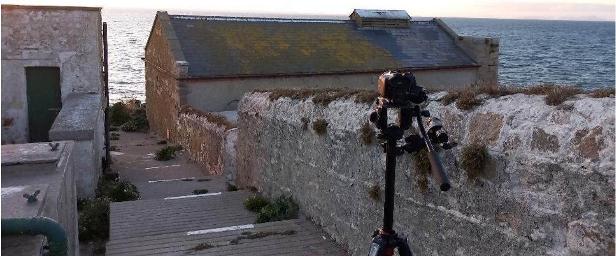
Plate 6: Building One, surveyor facing west/northwest
