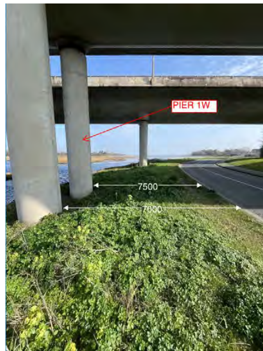
Figure 8 Carraigeway Offsets at Pier 1W
