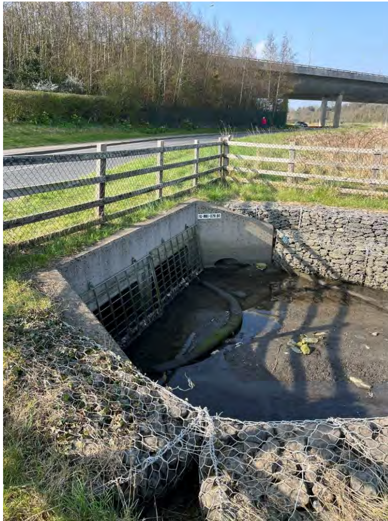
Figure 13 View of Wx-18 Crossing Location, facing North
